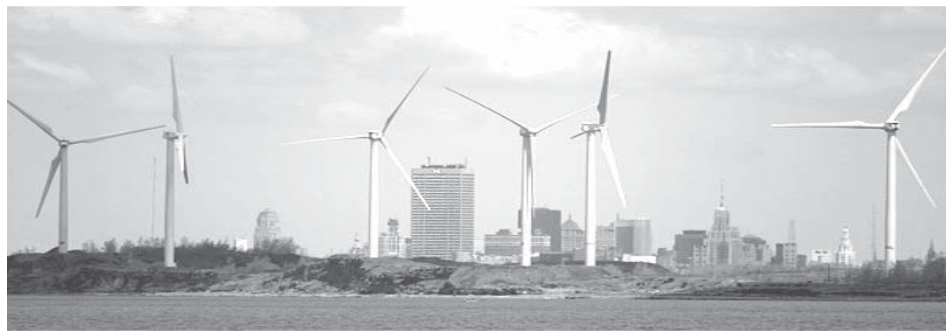
Eight large windmills at Steel Winds a former "brownfield" at the Bethlehem Steel site south of Buffalo, NY can power 7,000 homes. The 27 that are planned can light 23,625.
